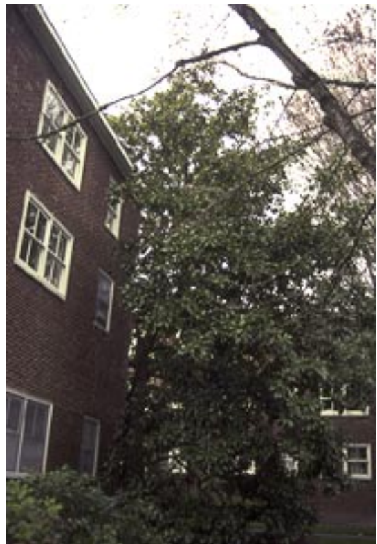
Figure 4. Vegetation allowed to grow too close to a building. May cause carpenter ant problems.
